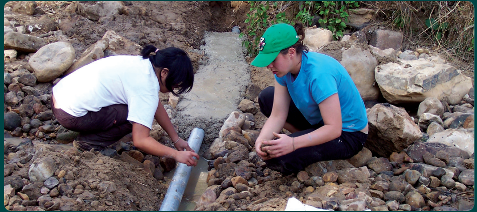
Engineers Without Borders student volunteers install a drainage pipe in Thailand.
